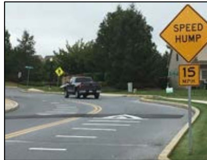
(Source: PennDOT Local Technical Assistance Program)
